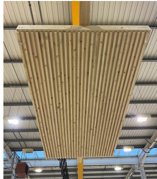
NLT Ceiling Panels (using beech nails)
